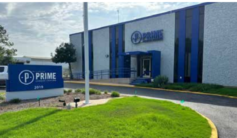
Prime Powder Coating's new Harbor Avenue location.
